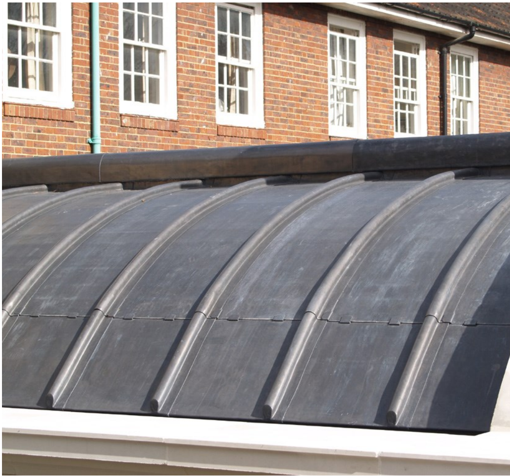
Lead sheet used for weatherproofing a roof
