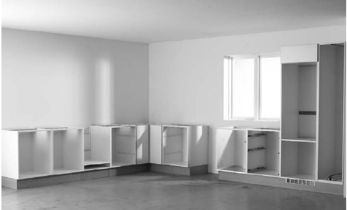
Melamine coated chipboard used in the kitchen cabinets and work surfaces
