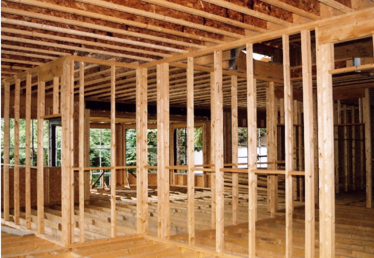
Red pine timber framing before being covered with plasterboard to form house walls and ceilings
