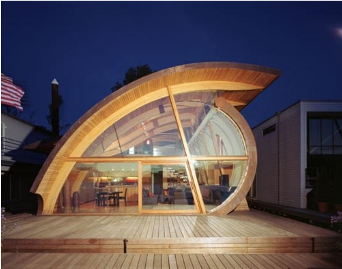
Glue-lam steam bent roofing beam in red pine
