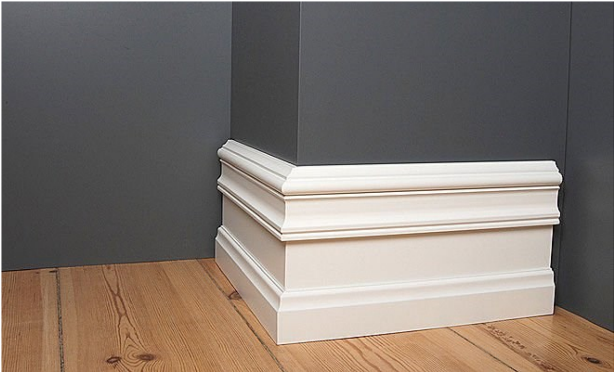
MDF skirting board - standard lengths machined on a spindle moulder
