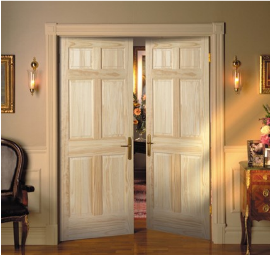
Moulded hardboard door skin over a pine frame finished to look like a solid timber panelled door
