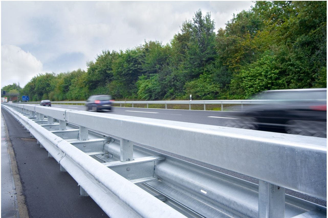
Galvanized steel crash barrier - bolted together to enable damaged sections to be replaced
